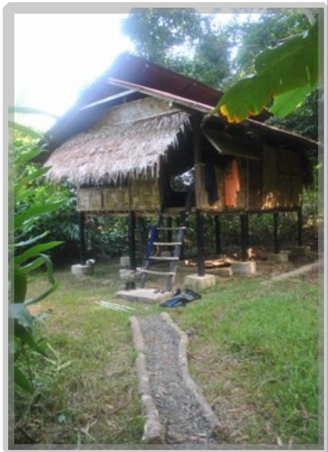
▲ Thatch accommodation at ANET
