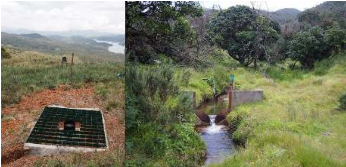
Figure 3-1: An example of a rain gauge installation (left) and headwater stream gauge (right) within our network in the Nilgiris area of the Western Ghats.
