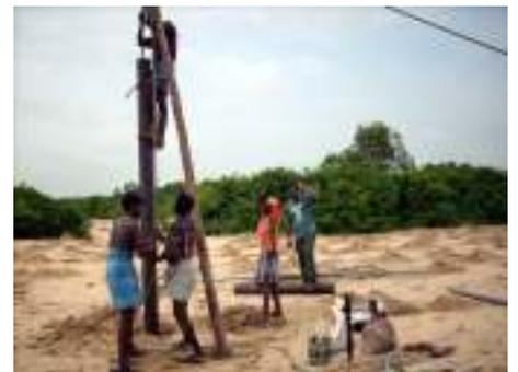
**Figure 6:** A manually operated auger well being used to drill shallow wells for a ecological restoration project in South India. Photo credits: FERAL.
