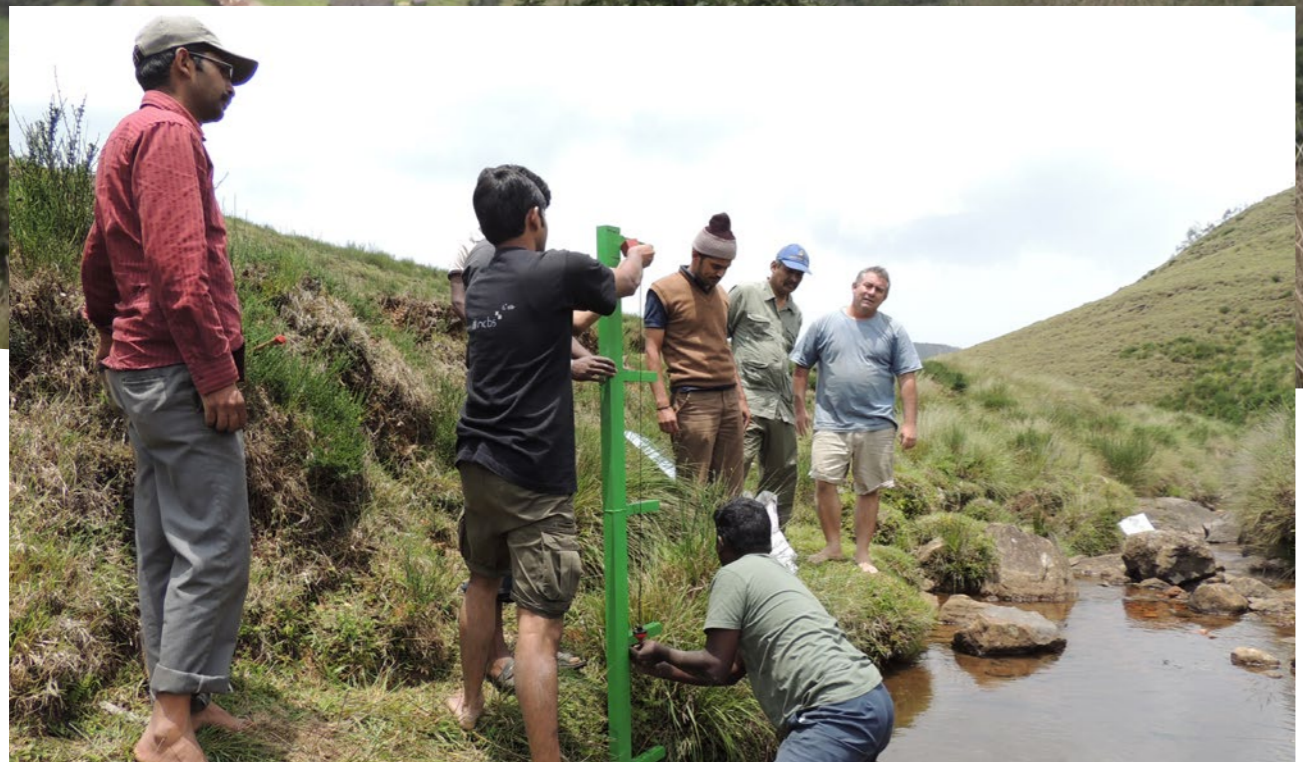
View of the Avalanche reservoir from the rain guage installed at the valve house. Below: Installing a water level recorder at the "bunker"
