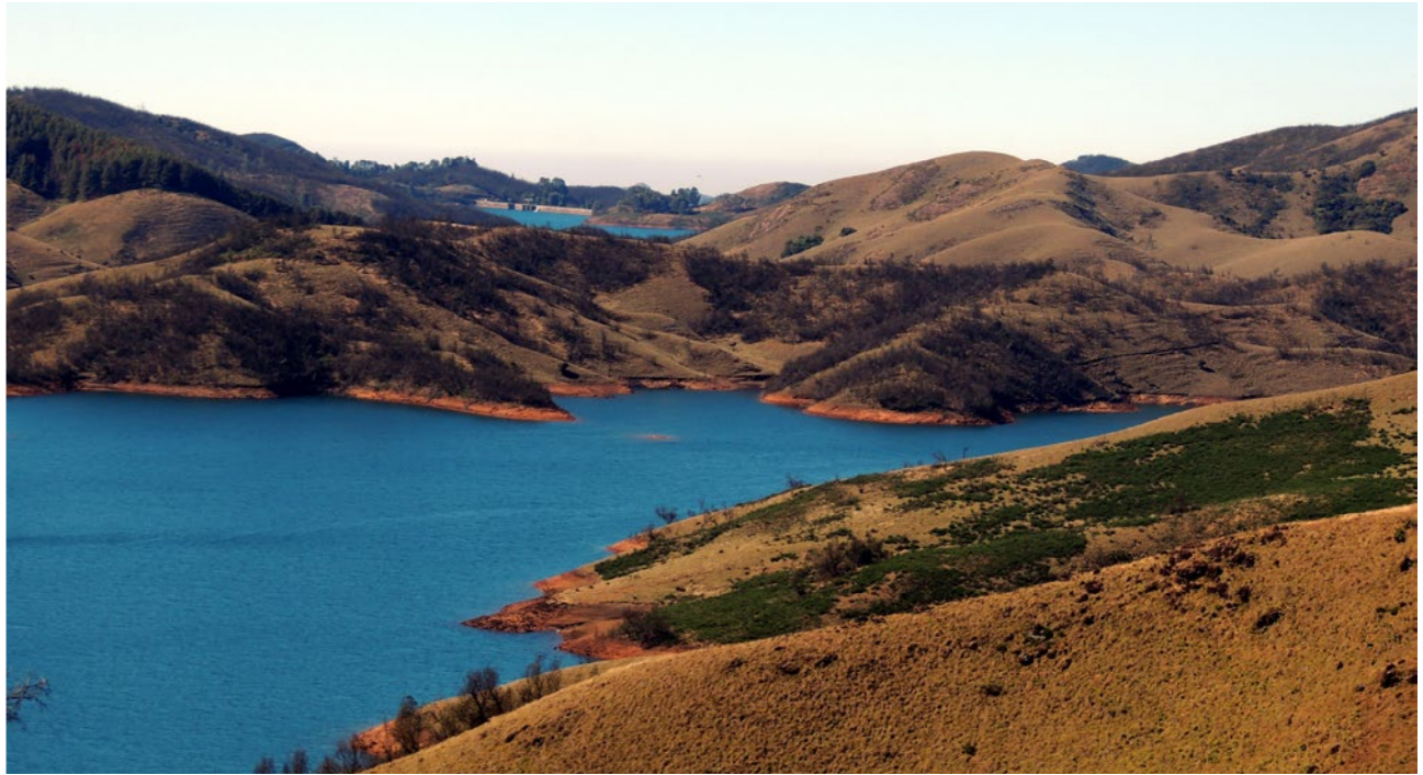
The Upper Bhavani dam benefits from the natural Shola habitat of forests and grasslands which sustain flows and filter out sediments from runoff.
