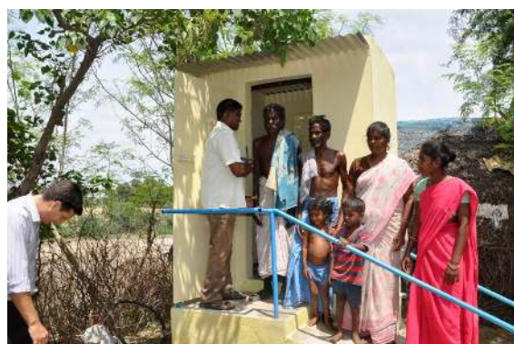
A newly constructed ecological sanitation toilet.
