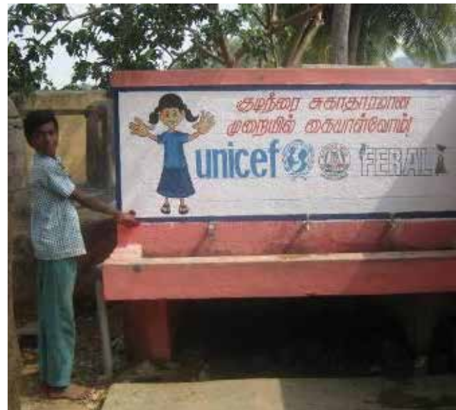
Fully repaired washbasin with new taps.
