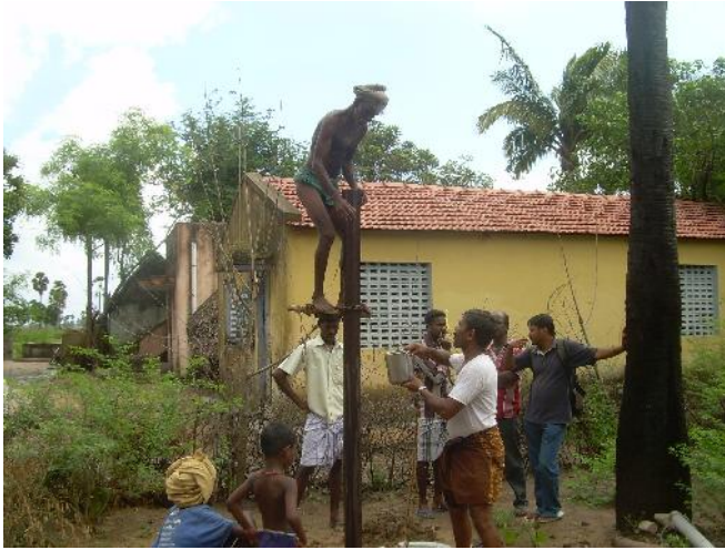
Figure 5.1.: A manually operated drilling apparatus in use.
