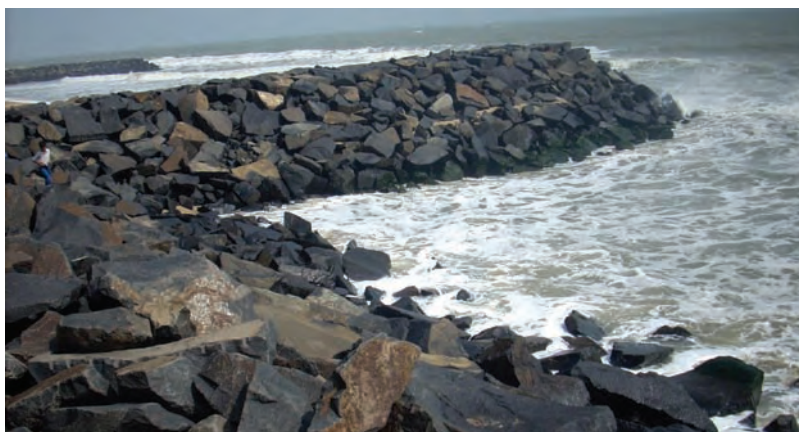
Figure 2.14: Groynes constructed along and to the North of the Pondicherry coast.
